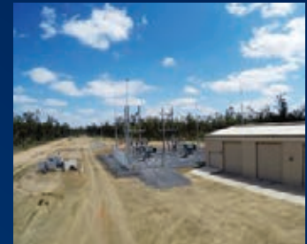
BINGEGANG PIPELINE RELOCATION MIDDLEMOUNT, QLD MIDDLEMOUNT COAL PTY LTD
